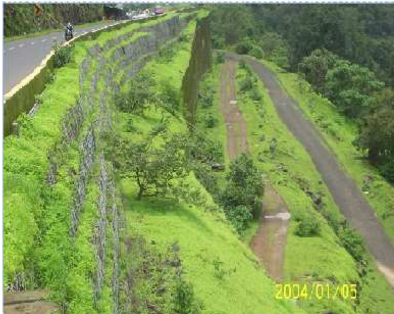
Gabion Wall for Mumbai-Pune Express way
